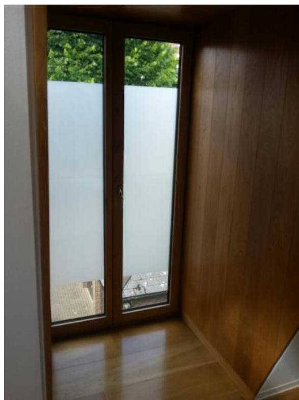
Front elevation (top) and view from within bedroom with obscured doors shut (bottom).
