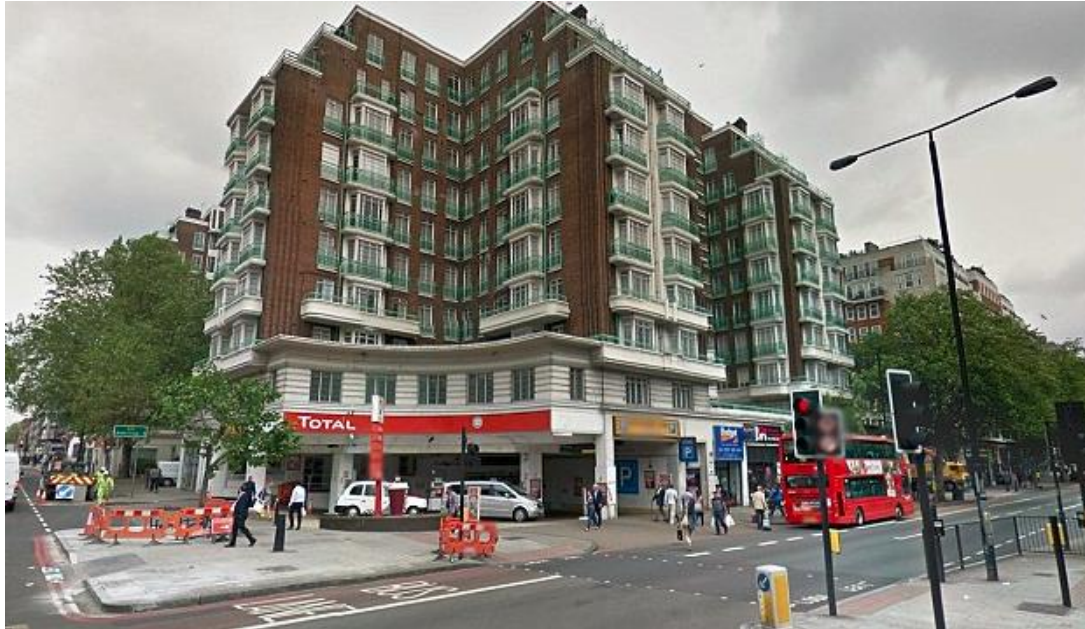
Dorset House, as seen from Marylebone Road with petrol station undergoing works (top) and prior to the fire in the underground car park (bottom).
